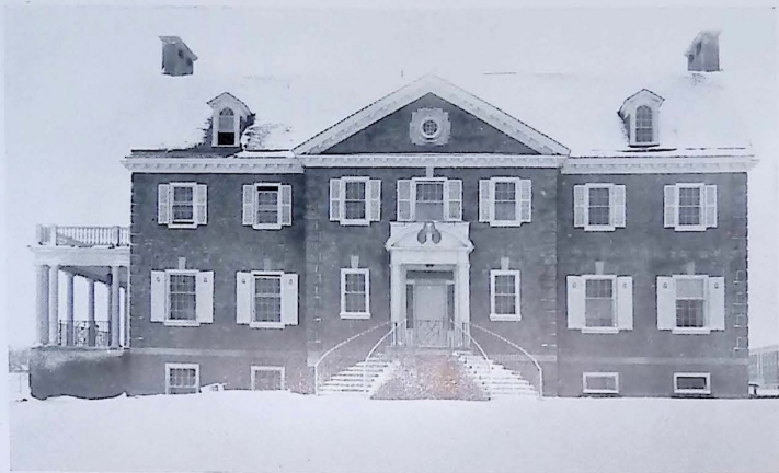
THE CHI HOUSE FACES THE WEST. THE RIVER IS JUST BACK OF THE PHOTOGRAPHER AND CURVES SO THAT THE PORCH ON THE NORTH END OVERLOOKS IT.
