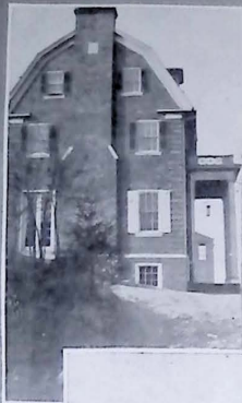
EAST END OF HOUSE
