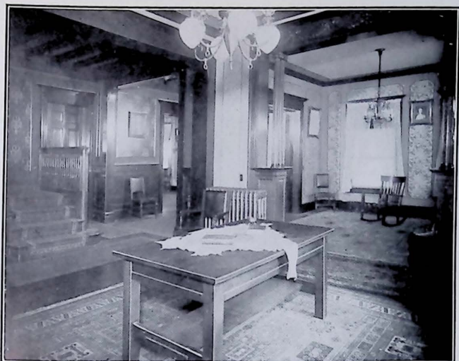
Looking from Lounging Room into Reception Room and Front Hall
