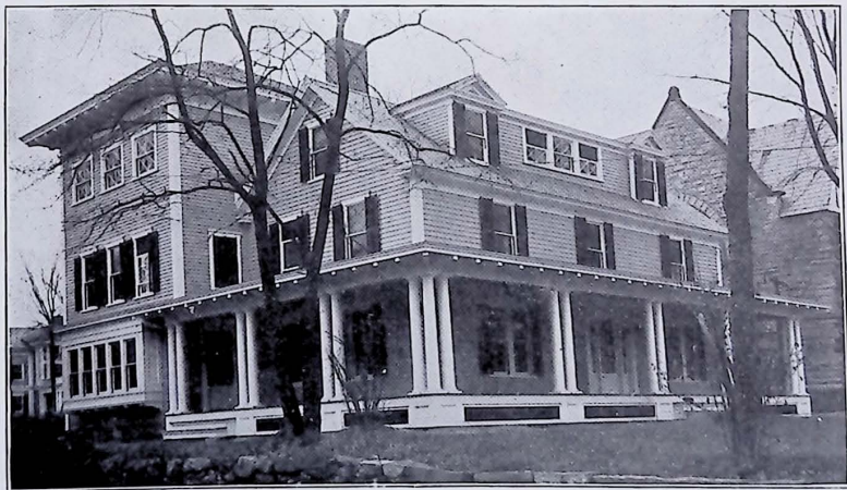
HOME OF 0 A ON WEST WHEELOCK STREET, HANOVER, N. H.
