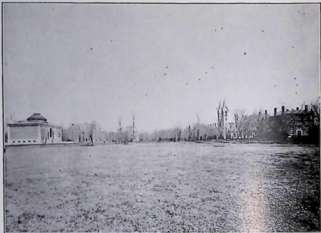
THE DELTA AND MEDICAL BUILDING.
